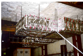
FyreWrap Elite 1.5 Fire Protection System For ADS
