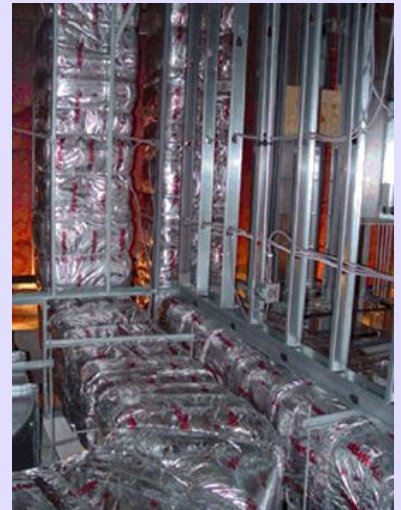
Typical FyreWrap Duct Wrap Fire Protection Application
